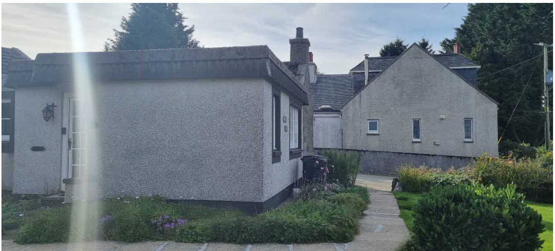
0148-01-PHOTO_002 (Flat roof Extension & neighbouring dormers)
