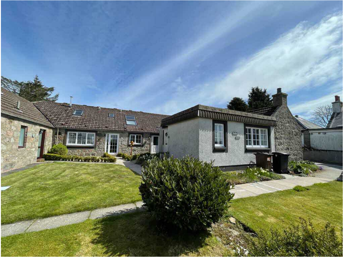
0148-01-PHOTO_001 (Roof extension & flat roof Extension)
